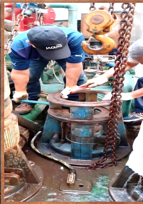
HEAVY-DUTY PUMP REPAIR AND LIFTING
