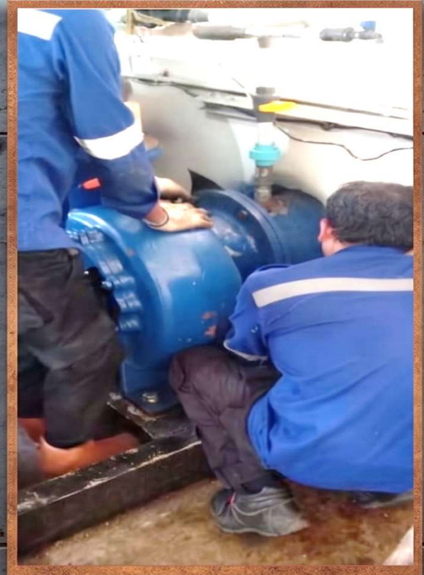
FINAL INSTALLATION AND IN-SITU TESTING
